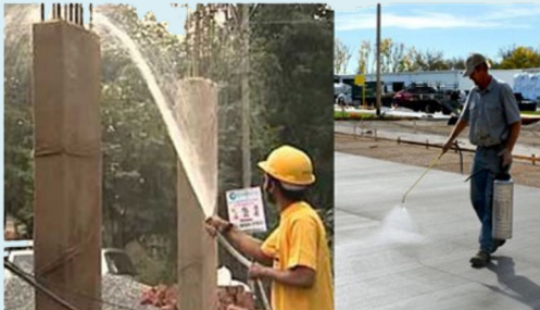
Fig E5.4 : Avoid large water force, use low pressure pumps for curing
