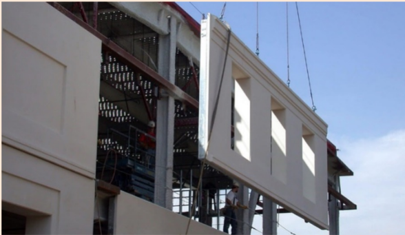
Fig B8.1: Precast walls for the exterior of the building
