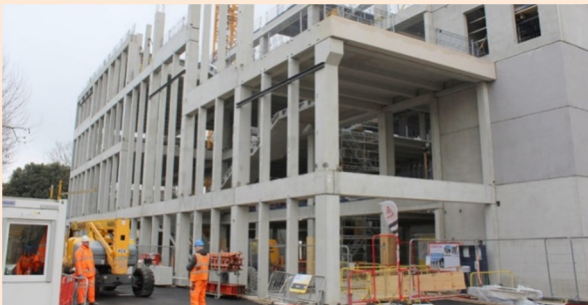
Fig B8.1: Precast beams and columns
