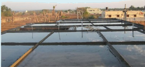
Fig E5.3 : Ponds made for curing on flat surface
